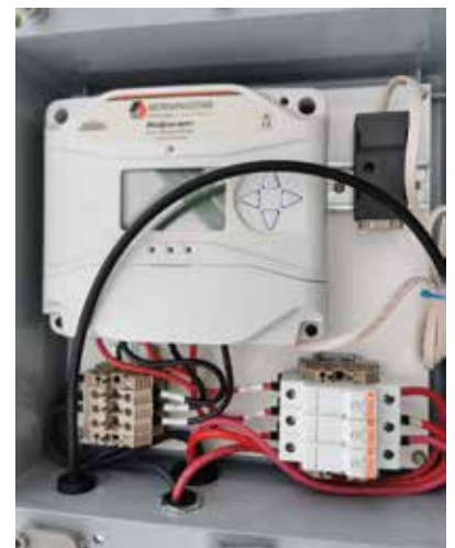
Morningstar ProStar MPPT 40M charge controller and MSC PC MeterBus Adapter
